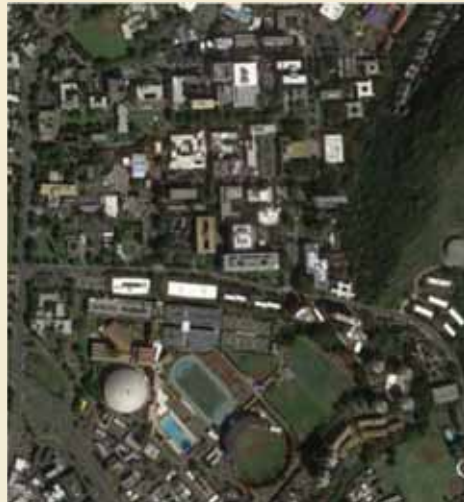
University of Hawaii – Mānoa Campus Microgrid
